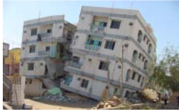
Figure 4: Typical collapse of RC Framed Building, 2001 Gujarat Earthquake
