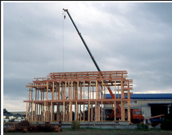
Fig. 5 Assembling members in building site
