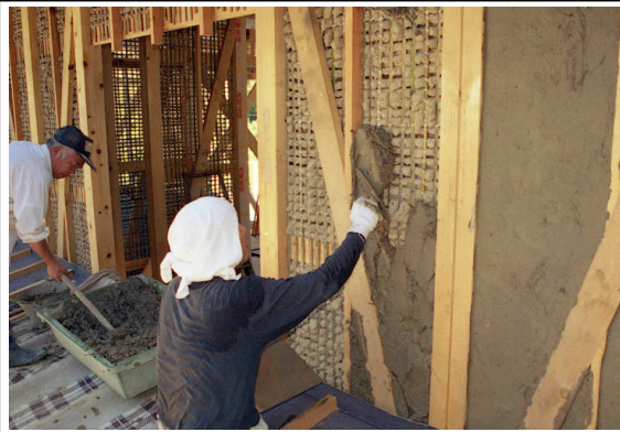
Fig. 11, Plastering Arakabe on bamboo lath
