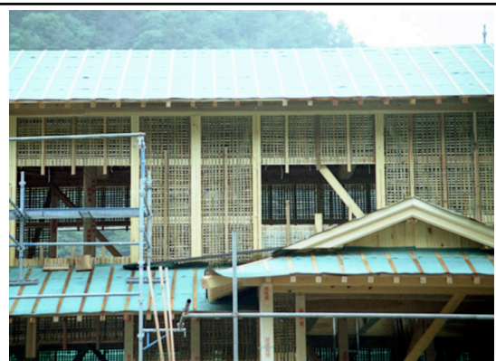
Fig. 10, Bamboo lath viewed from outside
