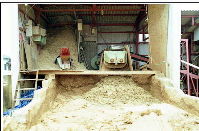
Fig. 7, Dorokon Plant in Toyohashi
