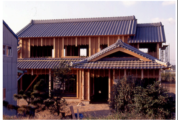
Fig. 14, Tile roofing completed
