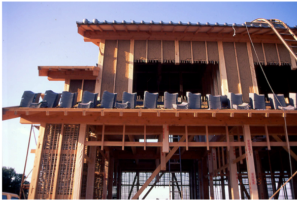
Fig. 13, Tile roofing in progress
