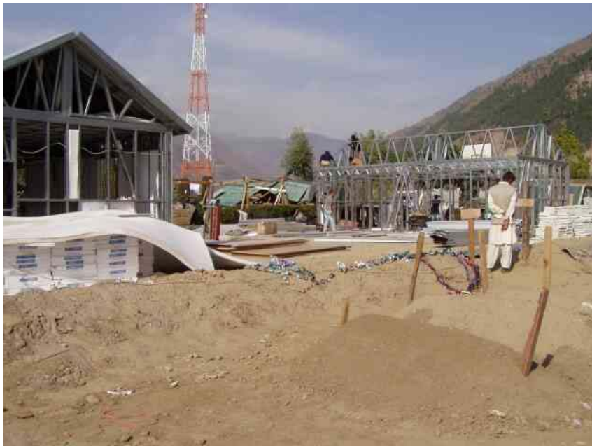
Collapsed School in Balakot, Pakistan
