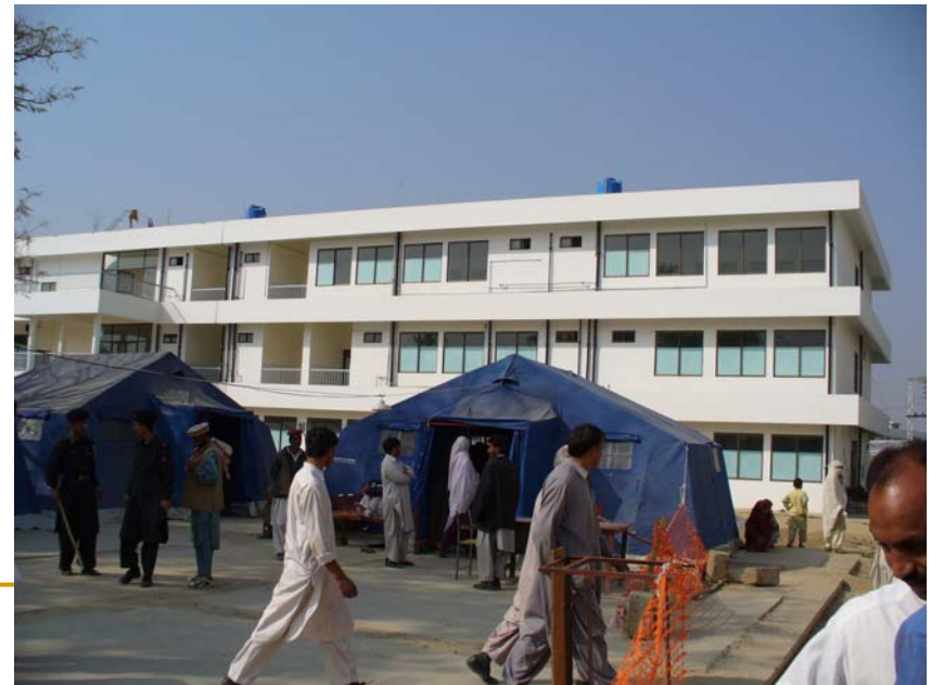
Damaged hospital in Mansehra, Pakistan
