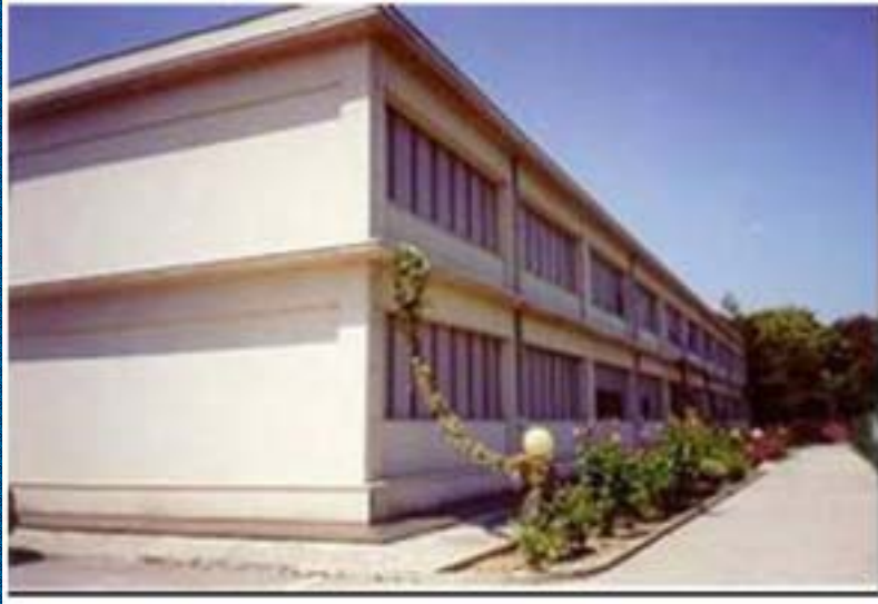
Training building for volunteers
