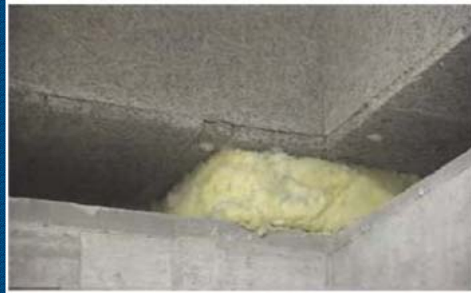
Fire protection of HDRB
