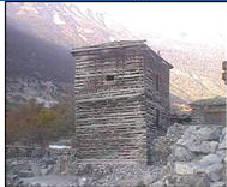
Figure 5 (b) A historical three story building, with single rooms at each floor, well standing the past seismic events.
