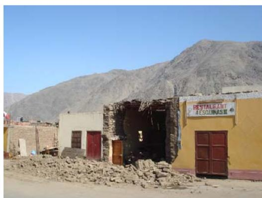
Photo 3 Adobe houses damaged by the Earthquake
