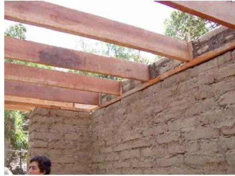
**Photo 9 Wooden roof beams (5x20cm) connecting**
