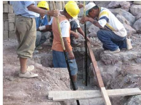
**Photo 5 Setting of vertical reinforcement
