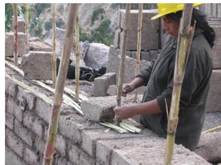
**Photo 7 Setting of horizontal reinforcement of crashed canes in every four layers connected to vertical reinforcement with nylon strings**
