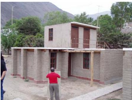
**Photo 4 Completed model house with many buttresses and raised foundation of concrete for prevention of humidity from ground (red pars H:30cm)**
