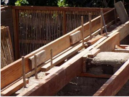
**Photo 8 Ring beams on top of adobe walls**
