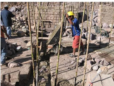
**Photo 6 Casting of concrete for foundation
