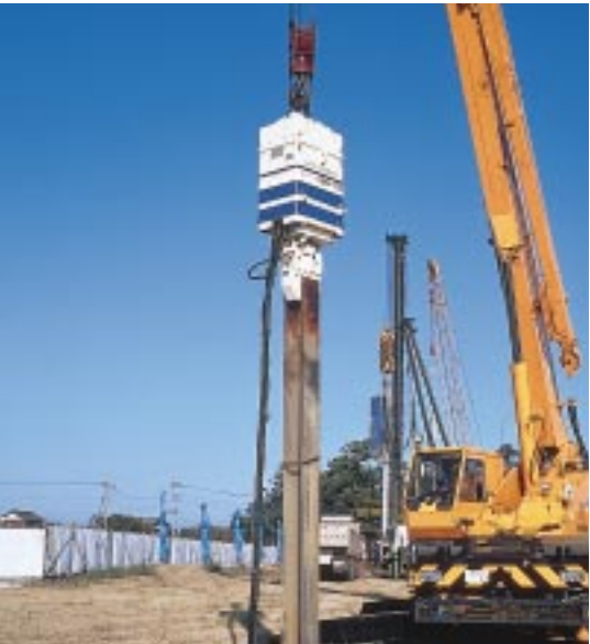
11. 建設工事環境改善技術の開発 地盤振動や騒音を抑える高周波杭打機 Development of technology for improving construction work environments High-frequency pile-driving machine designed to reduce ground vibration and noise.
