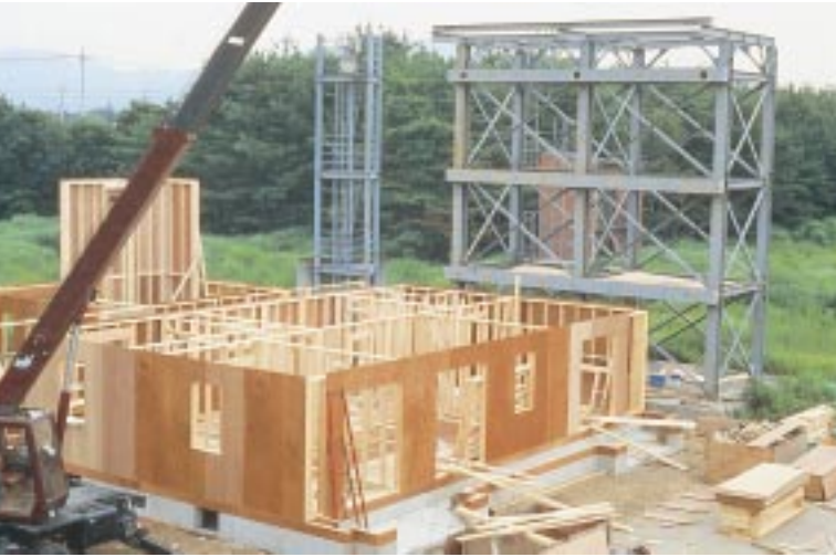
5. 小規模住宅新施工法の開発 2インチ×4インチの部材で壁と床板を作るツーバイフォー工法 Development of new construction methods for small-scale housing Wall and floor frameworks are built with dimensional timber ("two-by-fours").
