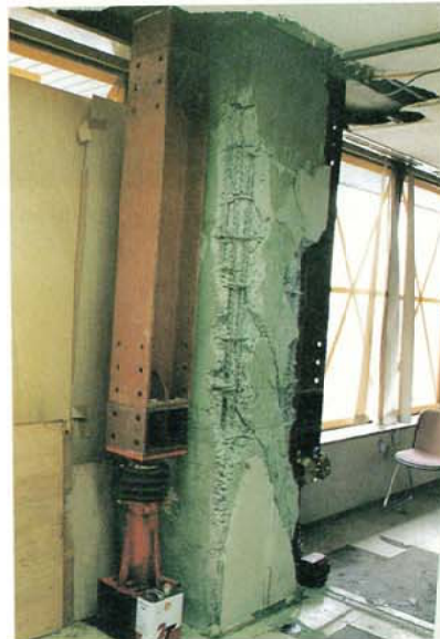
Photo . 3.2.1.62 Bond Splitting Failure of SRC Column
