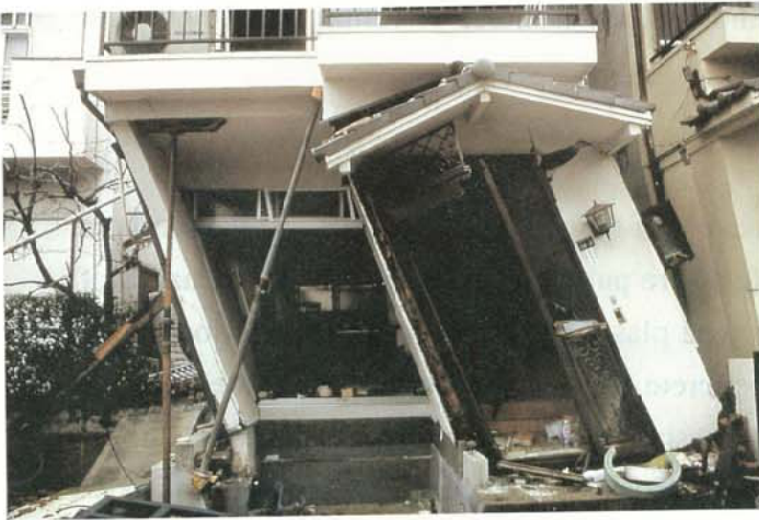
Photo 3.2.3.9 Wooden building with few shear walls
