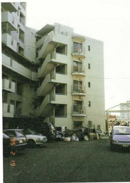
Photo. 3.2.1.57 South Facade of 5 Story Building
