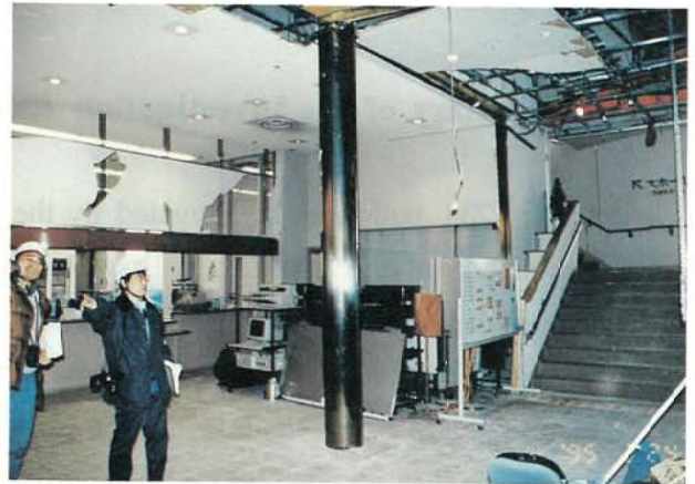
Photo 3.2.2.19 Damaged building interior due to pounding on parking building below (Building B)
