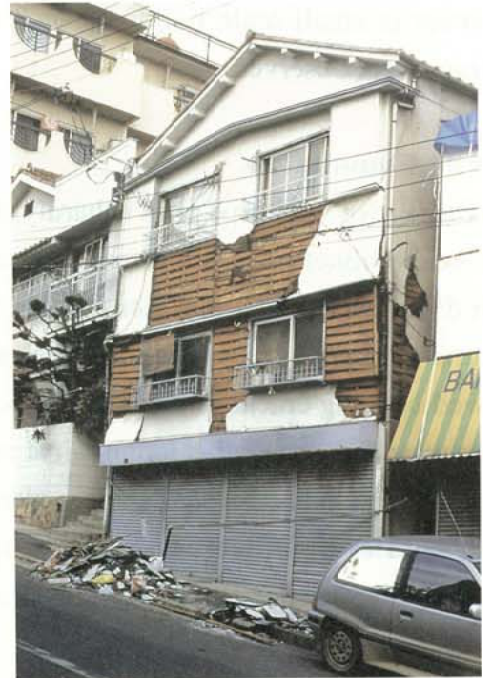
Photo 3.2.3.10 Damage of the exterior lath-mortar
