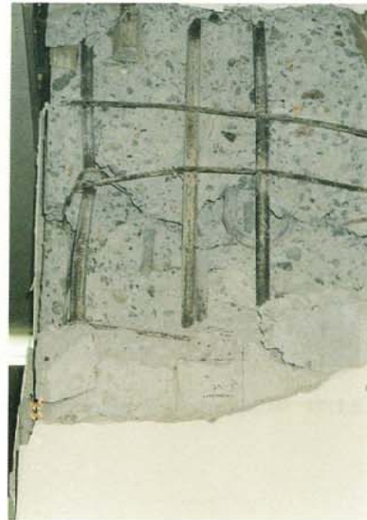
Photo.3.2.1.70 135degree hook in Reinforcement end
