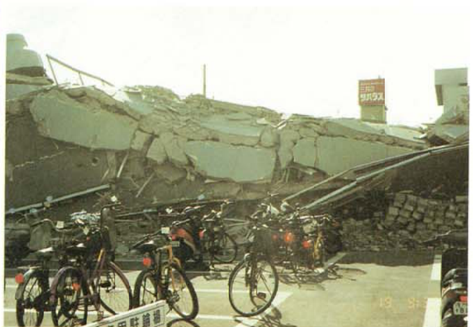
Photo. 3.2.1.28 Fracture in the form of a pan cake
