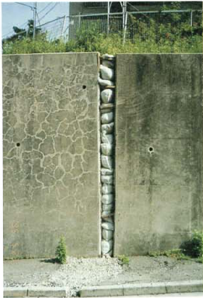
Photo. 3.2.1.11 Transfer of the breast wall (about 15cm)
