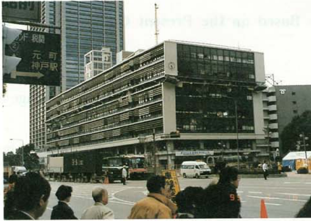
Photo.3.2.1.43 Total View ; The story collapse of the 6th floor
