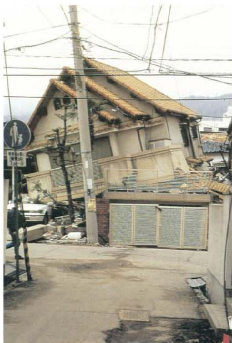
Photo 3.2.3.5 Collapse of the second story ( a garage of RC in the first story )
