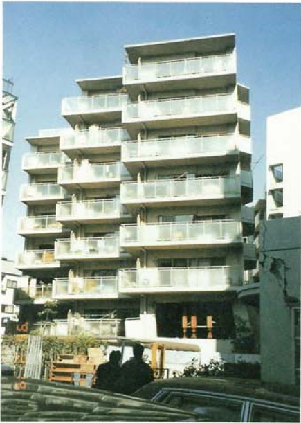
Photo. 3.2.1.49 South Facade of 8 story Apartment Housing
