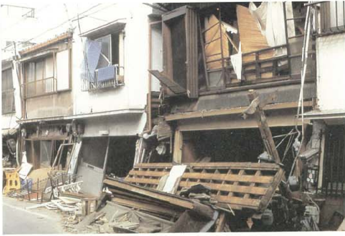
Photo 3.2.3.7 Building with a large opening
