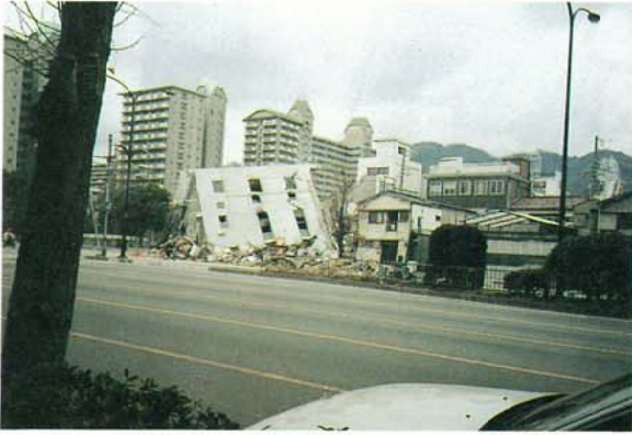
Photo.3.2.1.16 Overturning of the whole building
