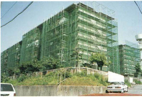
Photo.3.2.1.10 Total view of the building
