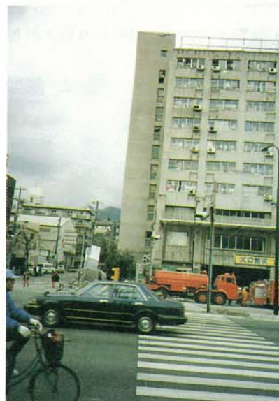
Photo.3.2.1.21 Fall of a penthouse
