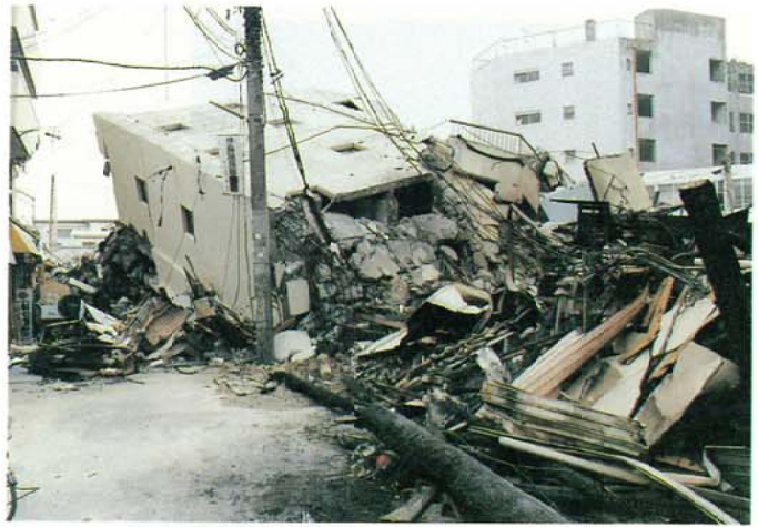
Photo. 3.2.1.17 Overturning of the whole building
