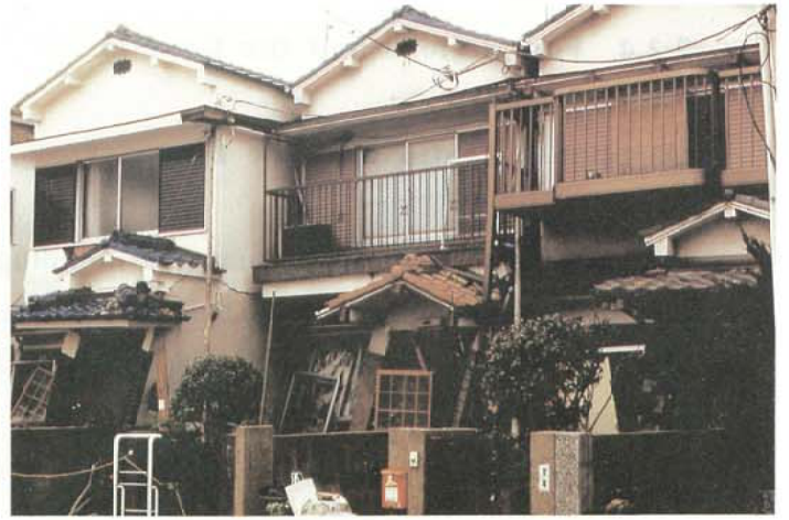
Photo 3.2.3.8 Wooden building with a small width
