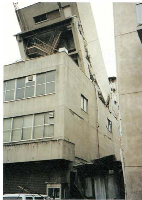
Photo. 3.2.1.23 Overturning of a penthouse
