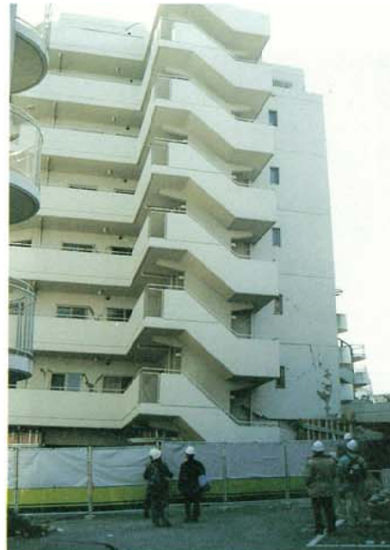
Photo. 3.2.1.50 North Facade ,Same Bldg.
