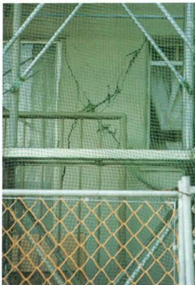
Photo. 3.2.1.12 Shear fracture creeping to the corners of the open part of the building ; windows & doors.
