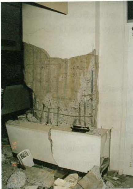
Photo.3.2.1.44 Basement ;Side column of the bearing wall column reinforcement
