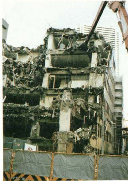
Photo . 3.2.1.59 Dismantling Condition of Building
