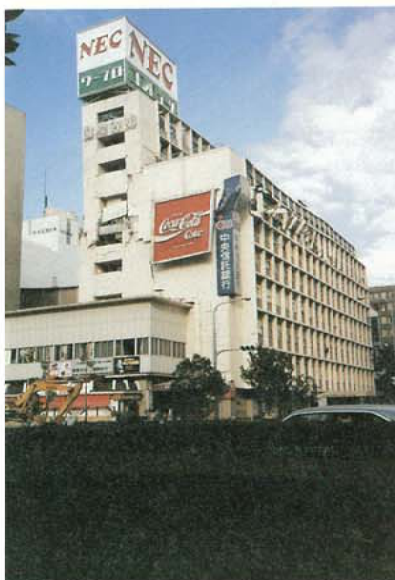
Photo. 3.2.1.24 Story collapse influenced by a set back
