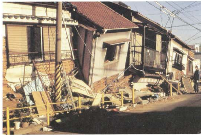
Photo 3.2.3.2 Collapse of the first story
