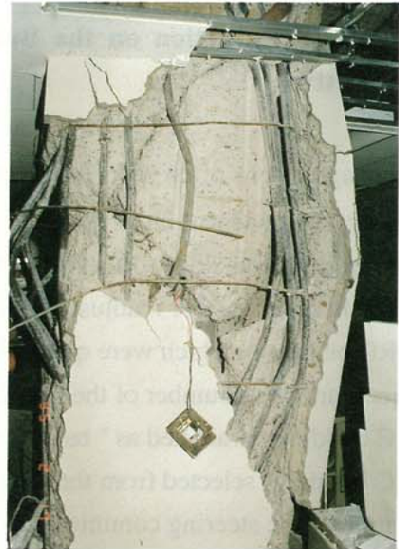
Photo. 3.2.1.46 Column of the 5th floor
