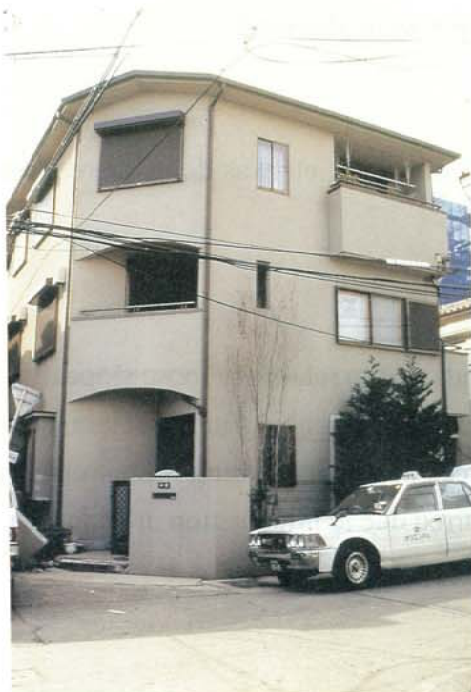
Photo 3.2.3.11 Three storey wooden building without damages
