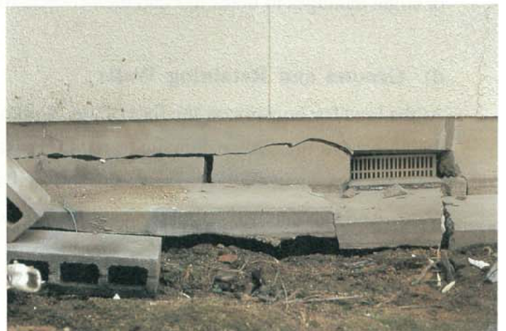
Photo 3.2.3.10 Damage of the exterior lath-mortar
