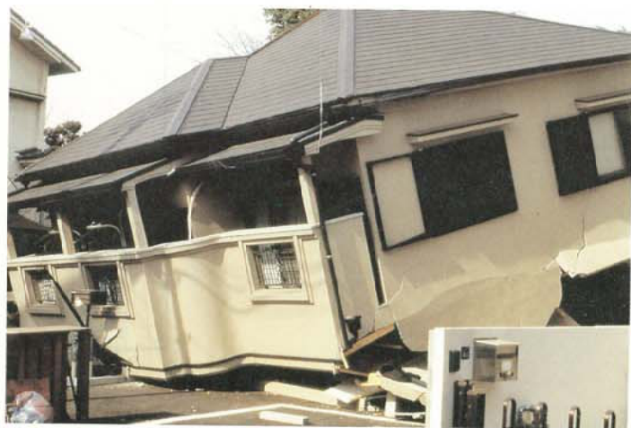
Photo 3.2.3.4 Collapse of the first story
