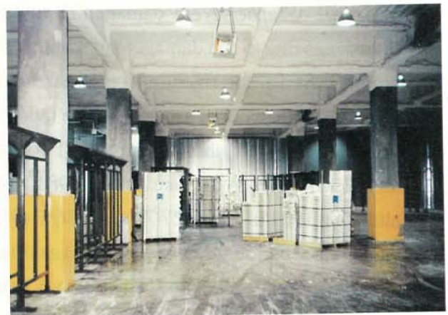
Photo 3.2.2.21 No damaged storage building (Building D)
