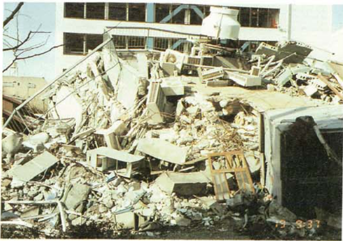
Photo. 3.2.1.27 Collapse in the form of a pan cake
