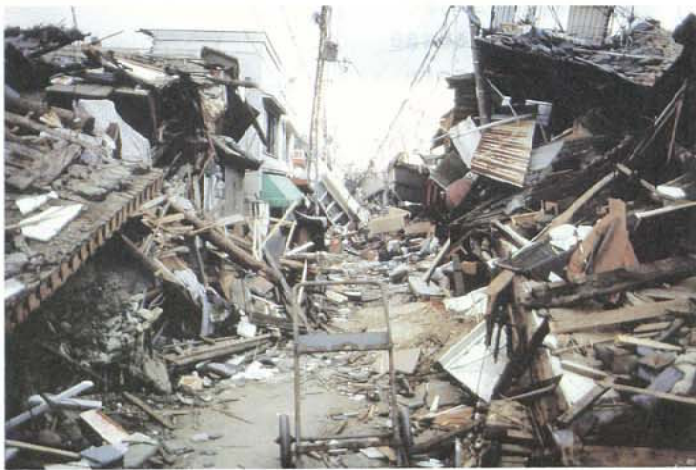
Photo 3.2.3.1 Collapse of wooden houses
