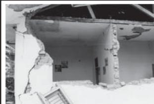
Damage to brick masonry, most of them have no reinforcement.
